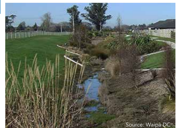
Stormwater reticulation culvert, Waipā
