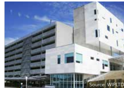
Meade Building Waikato Hospital, Hamilton
