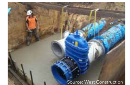
Water pipeline, Hamilton
