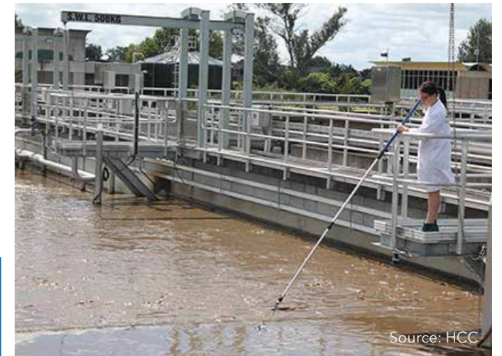
Wastewater treatment plant, Hamilton
